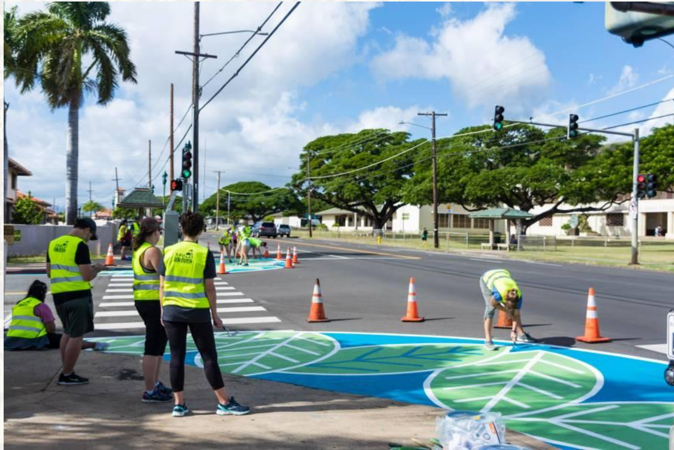
Volunteers finishing the Kalihi curb extensions across Farrington High School Photo credit: Ulupono Initiative From Justin Menina
